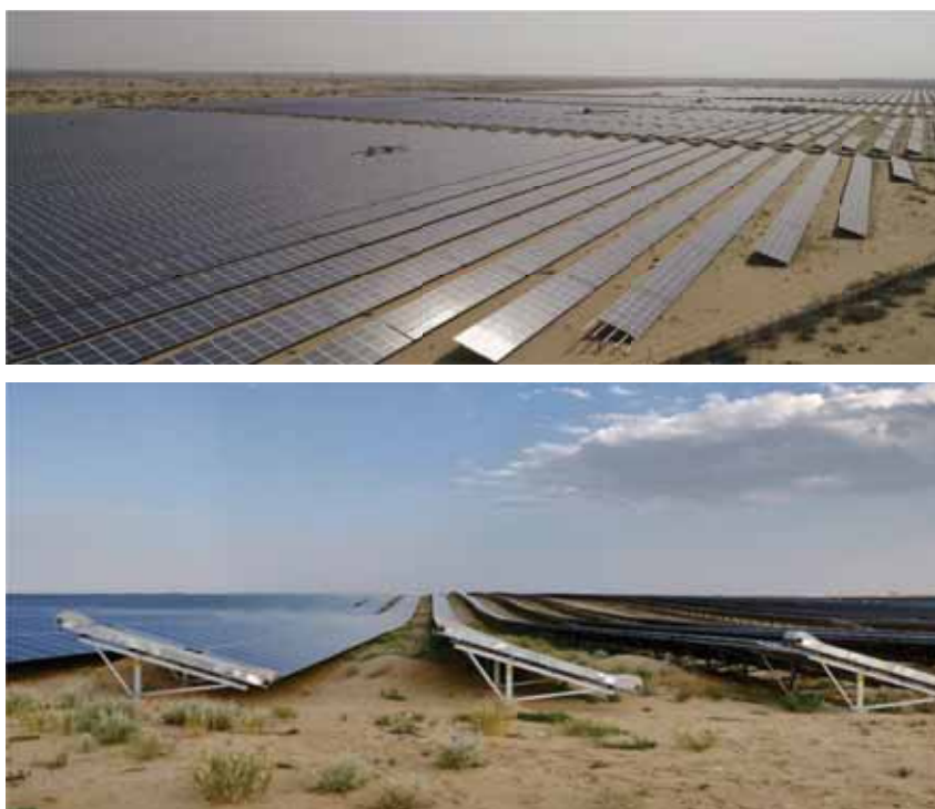
Figure 8 Solar projects inside solar park of Bhadla site
